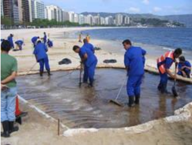
Figure 6.9 Flushing out oil buried in a sand beach using low pressure water supplied through lances and perforated pipes. Photo Credit: ITOPF; http://www.itopf.com/knowledge-resources/documents-guides/response-techniques/shoreline-clean-up-and-response/
